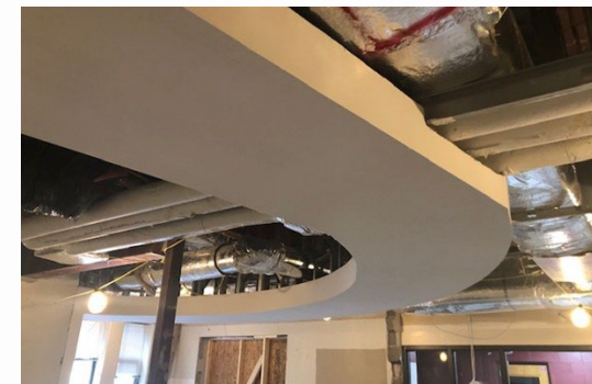
New Ceiling in Office
