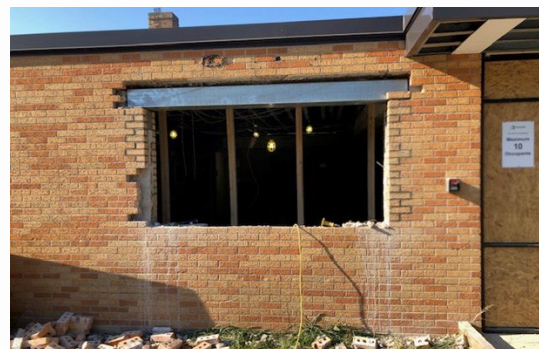
Creating Window for Office
