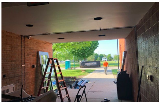
Removal of Old Entrance
