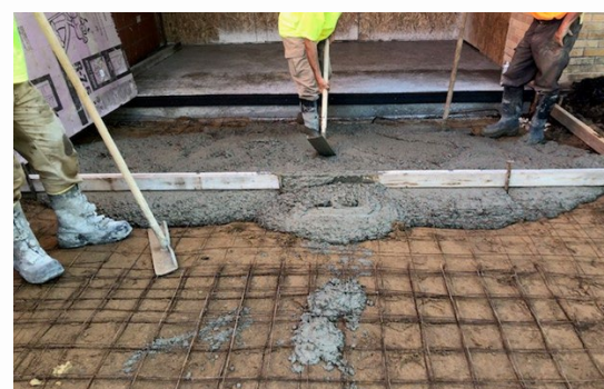
New Concrete Approach
